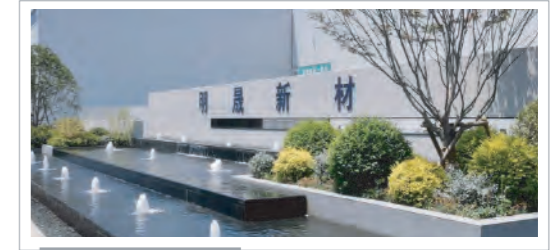
Henan Mingsheng New Materials Technology Co., Ltd. 30MWh Project
