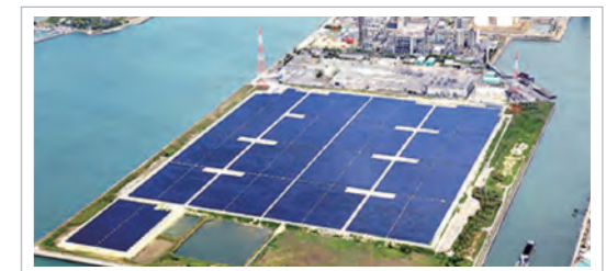
Japan UBE factory in Osaka 6MWh Project
