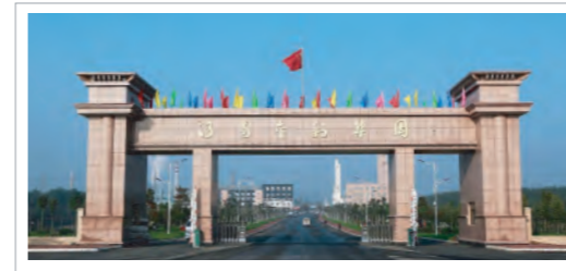
Henan Jinli Jin Lead Group Co., Ltd. 24MWh Project
