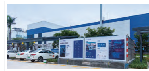
Guangdong Zhuhai 520kWh Solar-Storage-Charging Integrated Supercharging Station Project
