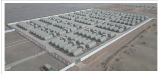
CNPC's Tarim Oilfield 600MWh Photovoltaic Power Generation Project
