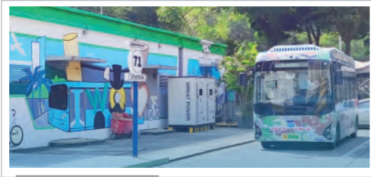
Shenzhen Bus Charging Station 60MWh Project
