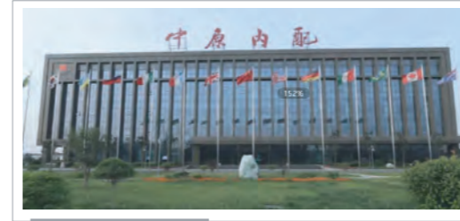
Henan Zhongyuan Internal Combustion Parts Co., Ltd. 40MWh Project
