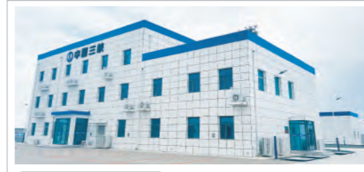
Ulanqab 180MWh Green Power Station Demonstration Project
