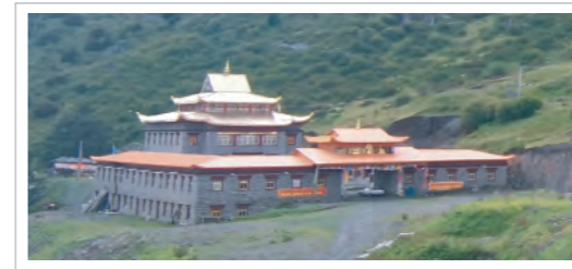
Kangding 392kWh Photovoltaic Off-grid Energy Storage Project
